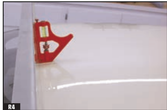
IT IS IMPORTANT TO HOLD THE TEMPLATE AT 90 DEGREES TO THE ROOF.
